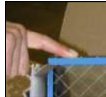
Glazing Tape is Pre-Applied to the Glass
