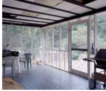
(Top and Above) Pictures taken of the porch before reconstruction show a dark, little-used area in poor condition. (Below) After the conversion to a sunroom, the homeowner gained bright, quiet spaces to read and view the outdoors.
