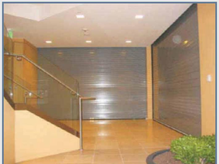
Temperature rise rated fire doors are required when used in exit enclosures or exit passageways
