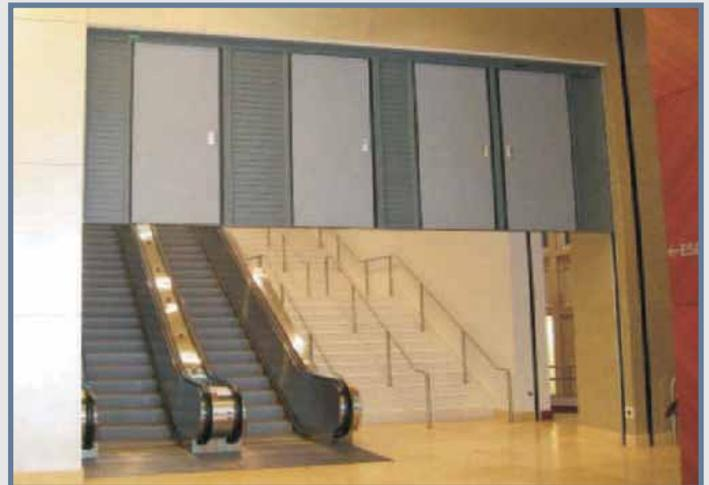
When activated, the fail-safe system lowers the coiling fire curtain and swinging emergency egress doors down into position....
