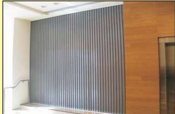
When activated, the fail-safe system begins to close without the aid of electricity or battery back-up.....creating the fire & smoke protection necessary for the opening.
