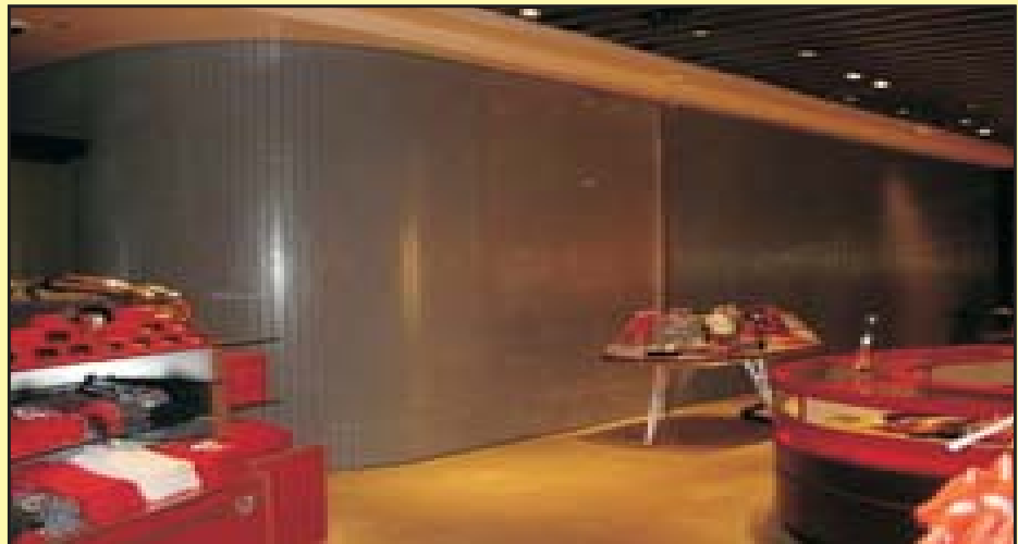
When activated, the fail-safe system begins to close without the aid of electricity or battery back-up.....creating the fire & smoke protection necessary for the opening.
