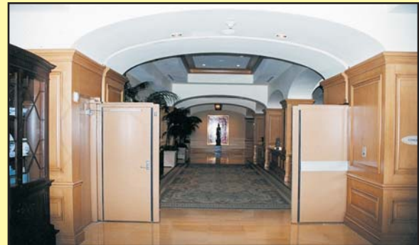
When activated hidden magnetic hold open devices automatically release emergency egress doors into position..
