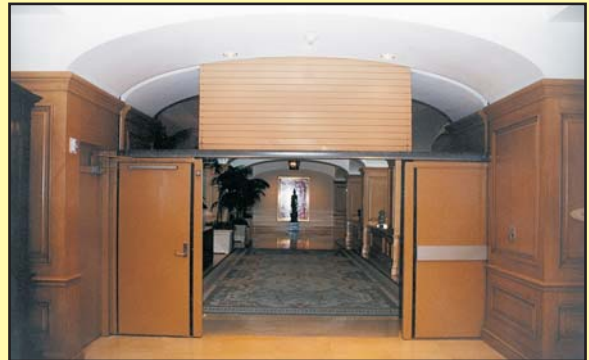
Within seconds, the fail-safe system lowers the coiling curtain into position without the aid of electricity or battery back-up...
