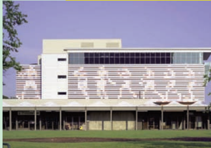
Muhammad Ali Center in Louisville, KY. Custom-colored KerAion Quadro facade panels form silhouettes.
