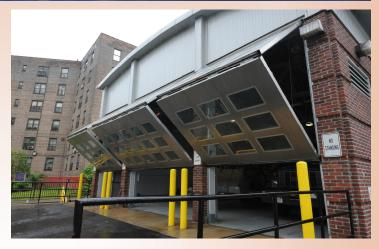
and providing reliable access in and out of the complex, is the facility three Wilson Premier  $^{TM}$  vertical bifolding doors. Two of the doors measure 10 øx 16 øto handle the heavy vehicle traffic and one door is for cars at 8 øx 16 øto
