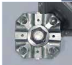
Panel engagement feature viewed from underside
