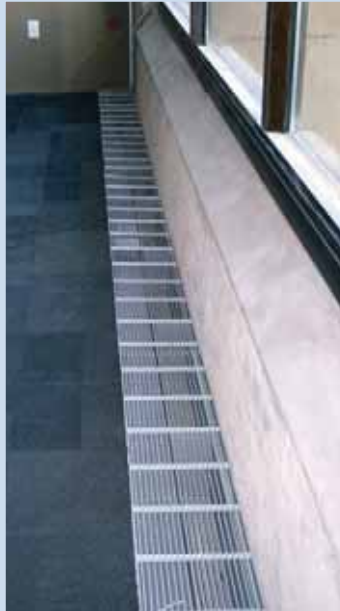
Active Chilled Beam for heating and cooling
