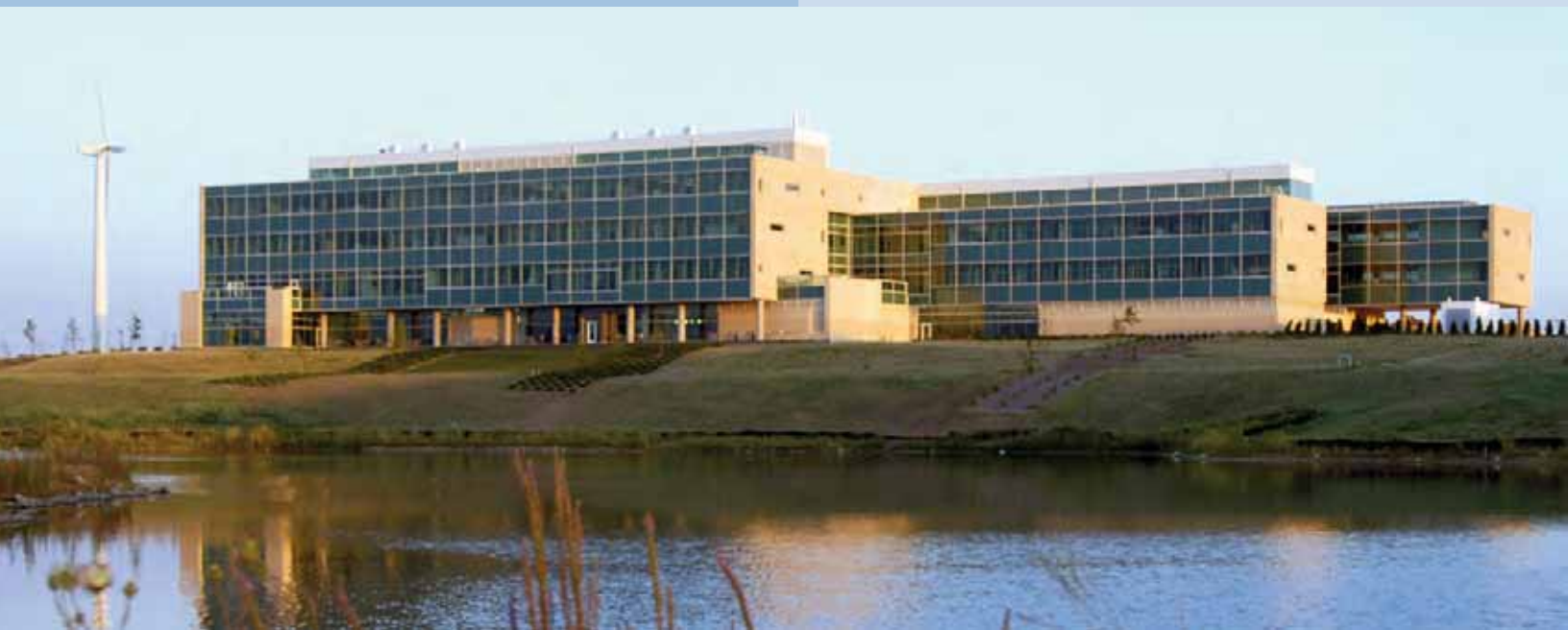
High Performance and Sustainable: Great River Energy, Maple Grove, MN, 166,000 ft 2 , LEED Platinum
