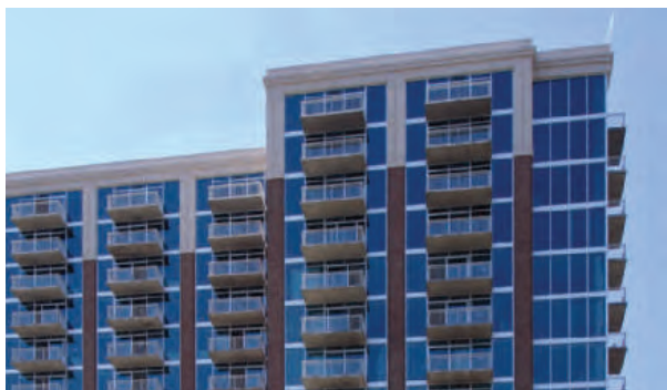
Vista on The James, Richmond, Virginia Architect: Rule Joy Trammell Architecture Glazing Contractor: American Door & Glass Systems Used: YCW 750 OG, YWW 50 T w/ slab edge cover, YSD 400, & Model 50D
