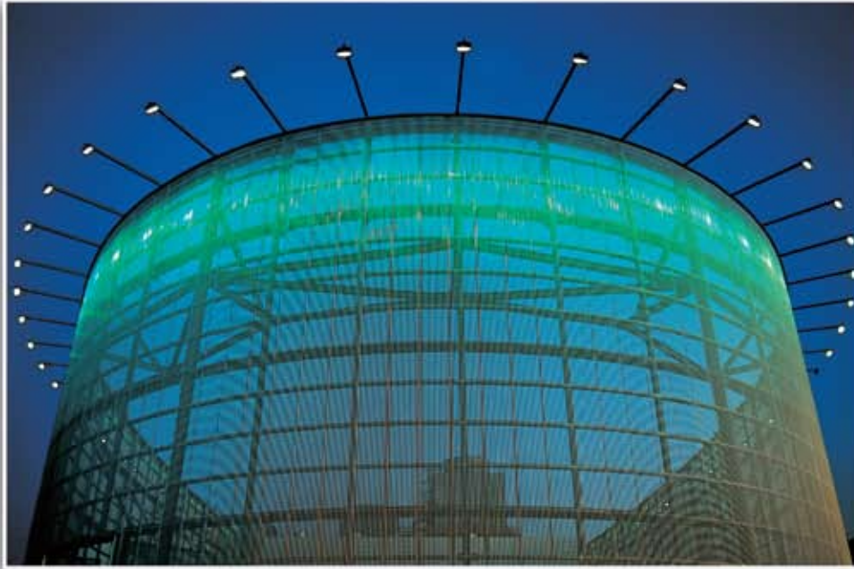
University of Pennsylvania Chilled Water Plant Philadelphia, PA
