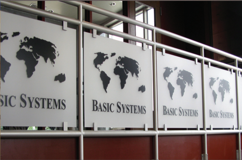
Basic Systems Cambridge, Ohio Railing Frame: Interna-Rail® Infill: Composite Finish: Clear Anodized Architect: Architectural Group – Cambridge, Ohio
