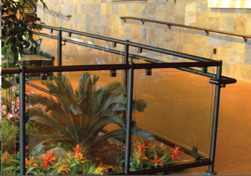
Choctaw Casino Choctaw Reservation, Oklahoma Railing Frame: Interna-Rail® Infill: Tempered Clear Glass Panels Finish: Dark bronze anodized
