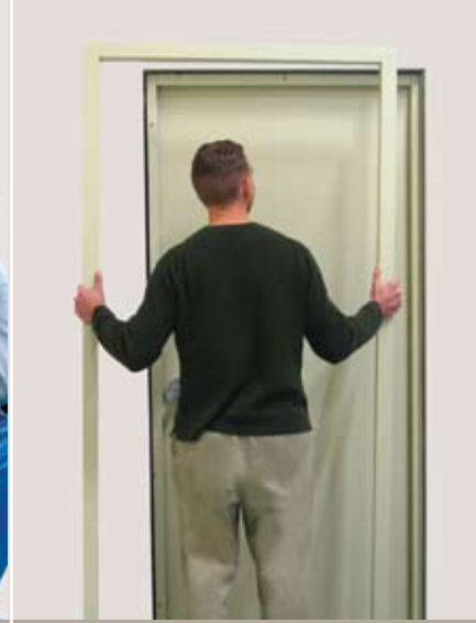
3. Frame trim piece is attached to unit and secured through the silencer holes – no exposed fasteners
