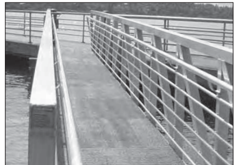
Fiberglass Grating was used to make a strong, slip resistant walkway for this outdoor setting.
