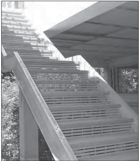
The Fiberglass Grating used for this stairway is well suited for an outdoor environment.
