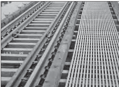
Pultruded T-Bar was easily field cut to make this corrosion resistant railroad walkway.
