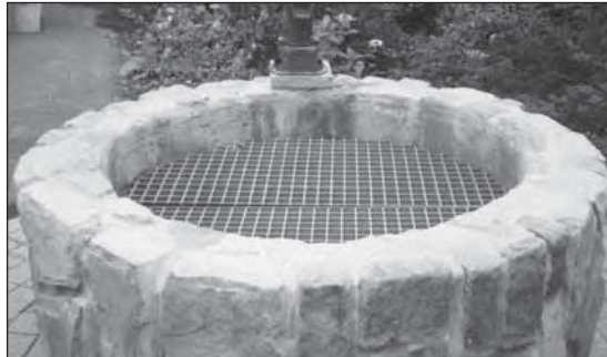
Square Molded Fiberglass Grating was used to make a cover to keep debris out of this stone well.
