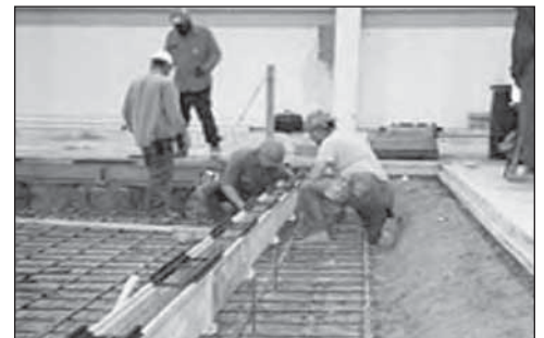
The installation/alignment chairs add to the ease of installing the trench drain system.
