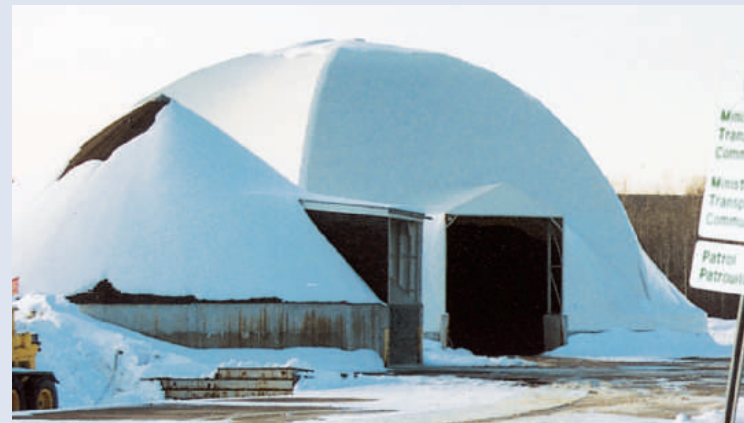
Sand/Salt Storage; Ontario, Canada
