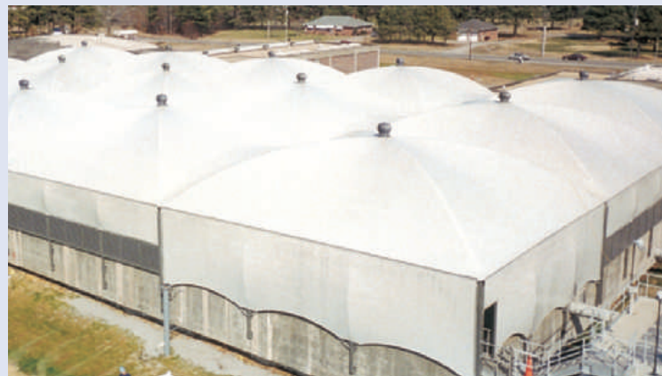
Water Treatment Facility; Chesapeake, VA
