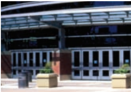
500 Tuffline® Entrances Ford Field, Detroit, Michigan Architect/Engineer of Record: SmithGroup, Detroit, Michigan Architects: Kaplan, McLaughlin, Diaz Architects, San Francisco, California; Hamilton Anderson Associates, Inc., Detroit, Michigan; Rossetti Associates Architects, Birmingham, Michigan Glazing Contractor: Universal Glass & Metals, Inc., Detroit, Michigan
