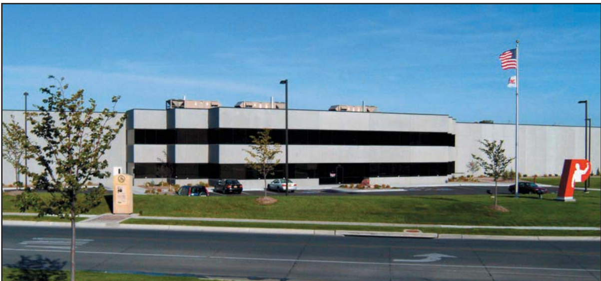
Headquarters and Plant / Omaha, Nebraska
