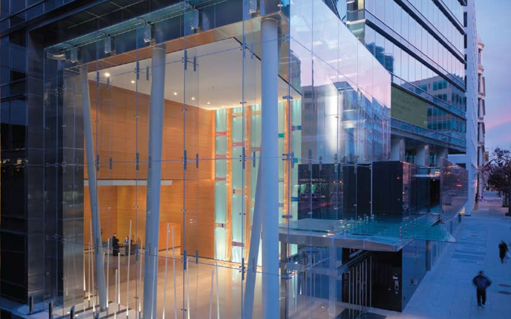
PROJECT Columbia Center
