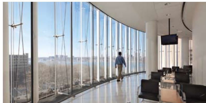
The exterior and interior facades are separated by a 3’ gap that accommodates both shading devices as well as stainless steel tension trusses for structural support
