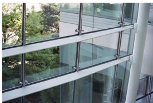
Horizontal painted steel plate beams resist wind load from the glazing and transfer it to the vertical steel jambs.
