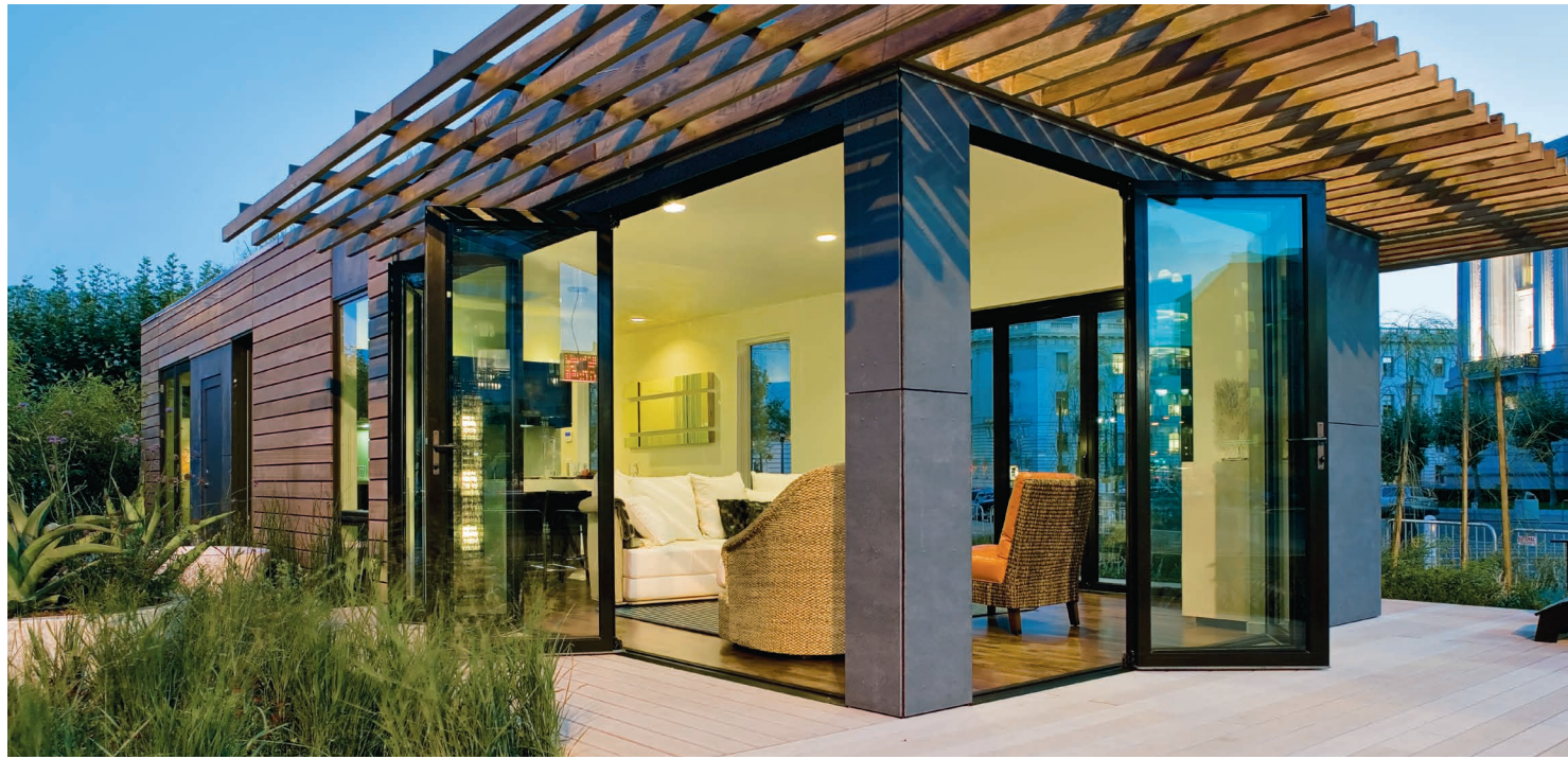
The mkLotus™ house features 12 operable glass panels of the NanaWall SL60.
