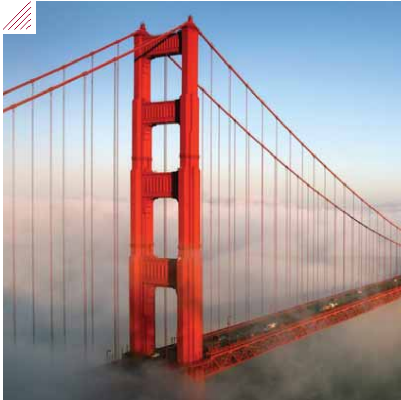
Golden Gate Bridge and Gate Operators - Municipalities
