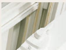
A precision-tuned **block and tackle counter balance system** on double-hung tilt windows makes lifting the sash a breeze and easily holds it open in any position.
